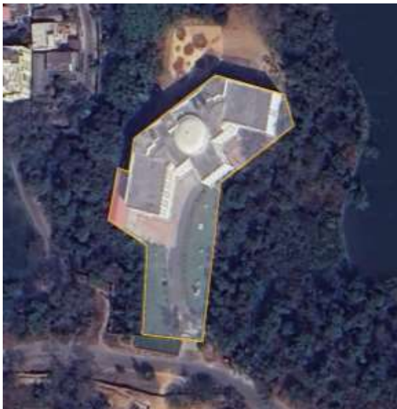
Figure 4: Area surveyed, Administrative Block
